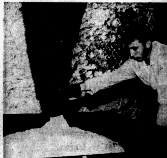
MASH MANIPULATOR — The ground-up apples, now a pulpy mash, fill trays which will soon be under the 90-ton pressure of the cider mill's ancient press. Bill Seldon, of Franklin Village, steers the mash into all corners of the wooden tray.
