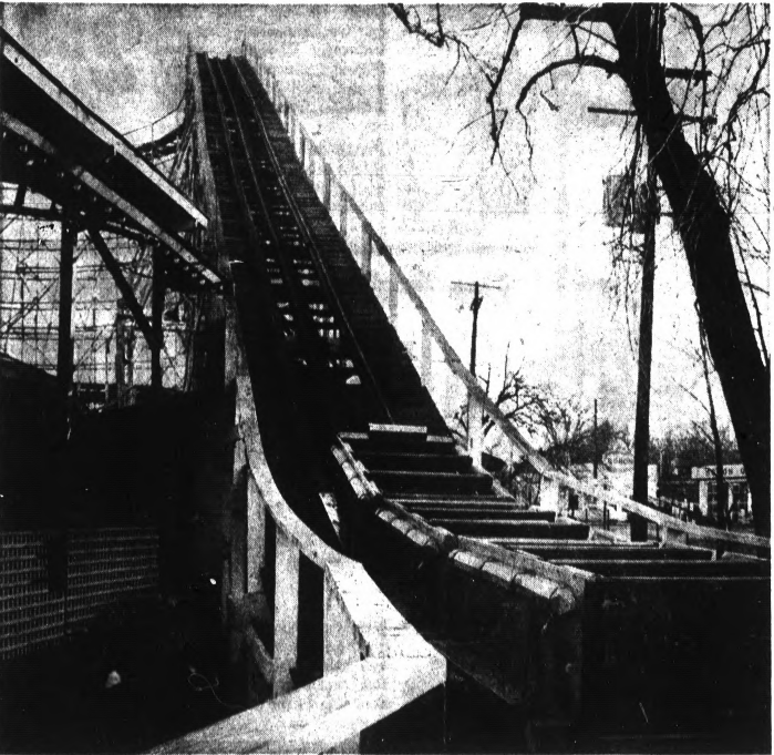
SLEEPING CARS — Resting after 40 years of hauling screaming children and stouthearted parents, cars of the once high-flying roller coaster now are idle on their siding at the former Walled Lake Amusement Park. They're awaiting their turn to be demolished by workmen now tearing down the Ferris wheel, the rocket ships and other rides in the park, which closed last September.
