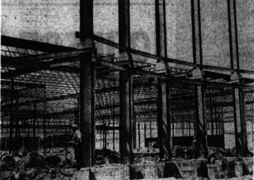
NEW MAIL PROGRESSING — Giant steel beams and a maze of smaller beams form the skeleton of the big mail at the Pontiac Mail Shopping Center on Telegraph at Elizabeth Lake roads. The construction picture changes daily as workmen pour concrete, transfer earth and erect beams for the new J. L. Hudson budget store and many other business places. The entire unit is expected to be in operation by next July.
