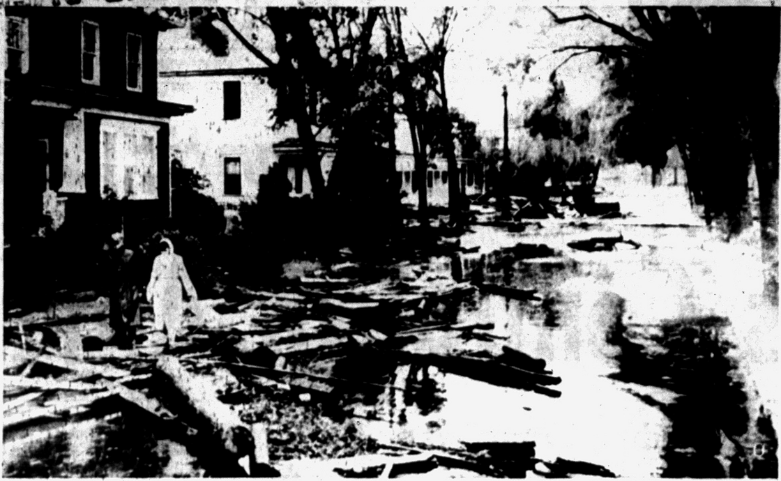
STORM WRECKAGE — Wreckage of houses blown down by hurricane Ione and washed about by flood waters clutter the streets near the New Bern, N. C., water front. Property damage is estimated to run into the millions.
