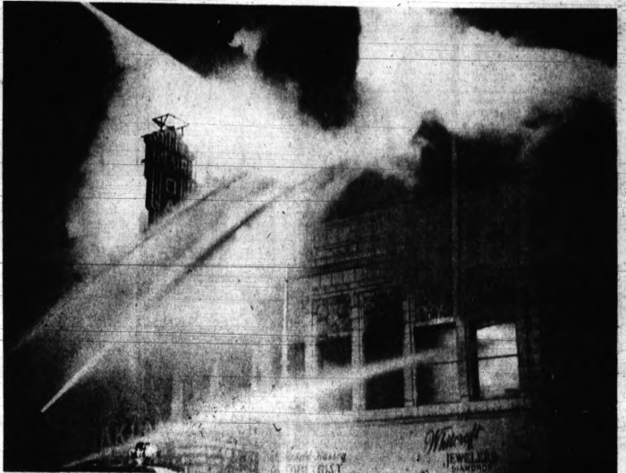
FIFTY-SIX EVACUATED — Fifty patrons and six employees were evacuated from the Oakland Theater on South Saginaw Street in time to escape flames that gutted the building. Firemen described the blaze as one of the city's worst. Over a hundred men
