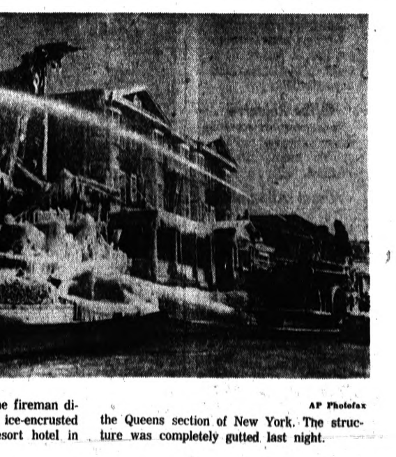
FIRE, COLD TOLL — A lone fireman directs a stream of water on the ice-encrusted ruins of the Far Rockaway resort hotel in the Queens section of New York. The structure was completely gutted last night.
