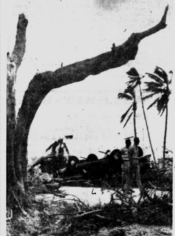
HAVOC OF NATURE — Broken trees and scattered tree limbs almost obscure two automobiles piled together by the winds in last night's tornado at Miami, Fla.
