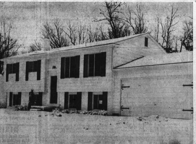
GOLF MANOR — The Smoker Co., builders and developers of many area subdivisions, are especially proud of the Berkley, in Golf Manor in the Union Lake area. Shown above, the $16,250 model is really a raised ranch house — a ranch house that has been pulled up out of the ground four feet. The living area is all
