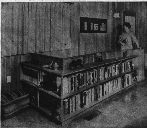
SHELVES FOR STAIRWELL — Here's a way to make the railing around the top of a stairwell an important, useful item. Low wall of tongue-and-groove western red cedar panels replaces usual open rail. Added book shelves take little space, contribute function and beauty.
