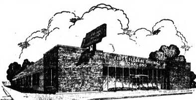
TELEPHONE: FEDERAL 3-7071 761 WEST HURON STREET
