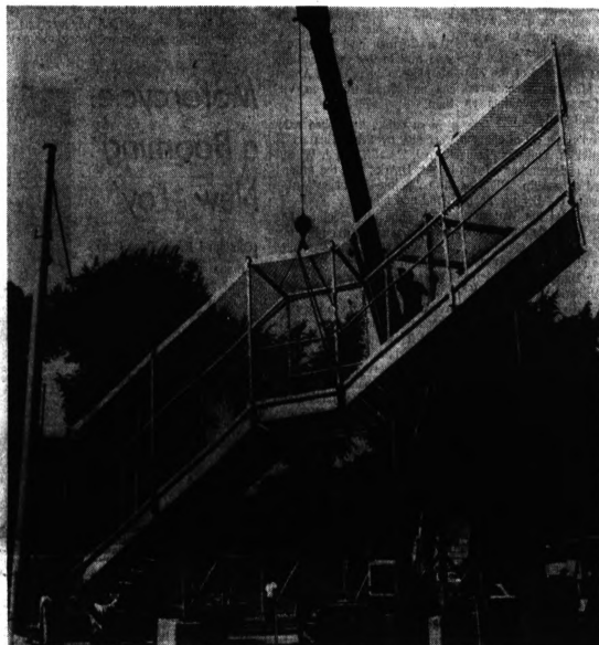
ERECT BRIDGE — Construction crews move the first section of the city's first pedestrian bridge into place on West Huron in front of Webster School. The boxlike span is the first of three
