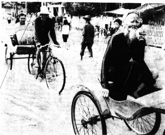
FLOODING HITS DELTA — South Vietnamese civilians move through the flooded streets of a Mekong Delta town in Chau Dox Province, near the Cambodian border. Floodwaters from heavy mon-
