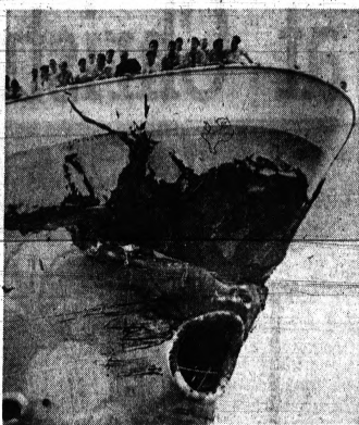
SHOW WOUNDS — Crewmen of the British luxury liner Oriana (left) and the aircraft carrier Kearsarge (right) look over the damage resulting from a collision of the two ships outside Long Beach, Calif. earlier this week. The carrier sustained
