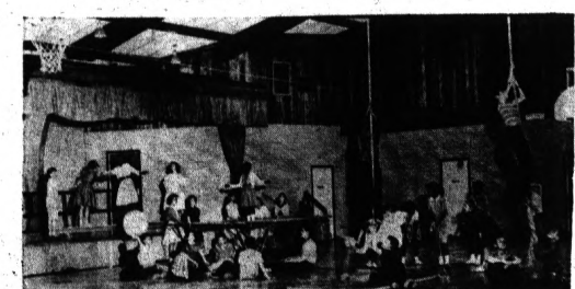
Multipurpose Room—Physical Training
