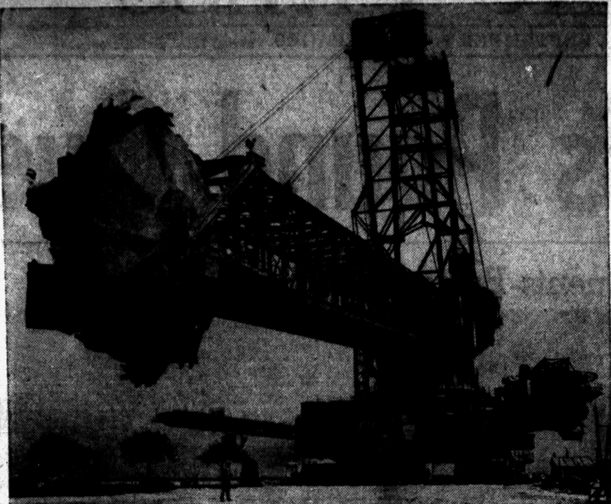
GIANT ON THE MOVE—This 6,000-ton dredging machine looms above the landscape at Duerwies, Germany, as it lumbers under its own power to a nearby job. The huge digger, built in two years, has an overall length of more than 500 feet and is over 200 feet high.
