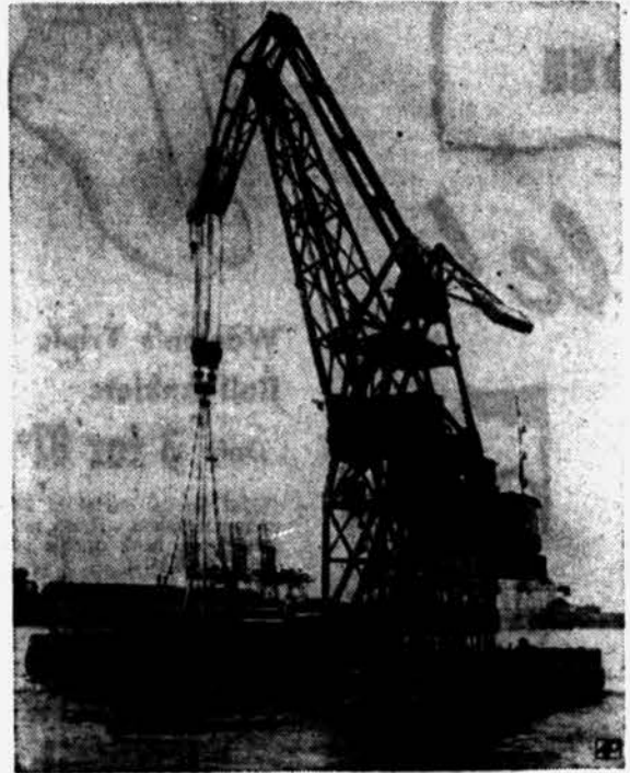
FLOATING POWER — Germany's largest floating crane goes to work in Hamburg harbor. The new hoist is powered by a 515-h.p. diesel engine and has a lifting power of 200 tons.
