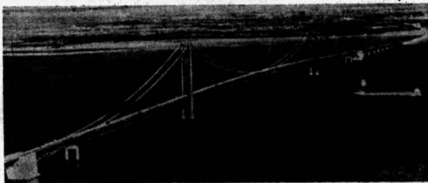
NEW MACKINAC STRAITS BRIDGE — The span is a boon to tourists heading for Northern Michigan. The bridge joins Lower and Upper Michigan at Mackinaw City and St. Ignace, linking the state's two peninsulas by land for the first time.
