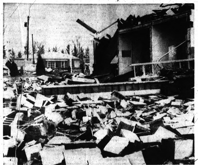
AP Wirephoto TWISTER DEBRIS IN OWOSSO — The roof and much of the contents of this Owosso gasoline station were lifted up and deposited across the street when a tornado struck shortly before midnight last night.
