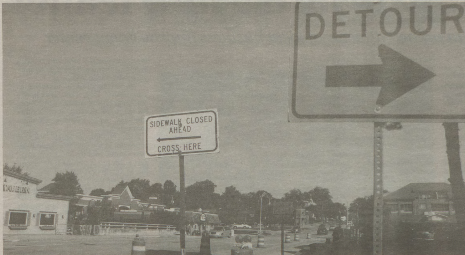
Work in Rochester lasted one construction season, from April to December. Projects included sidewalks, roads and bridge work, among other renovations.
