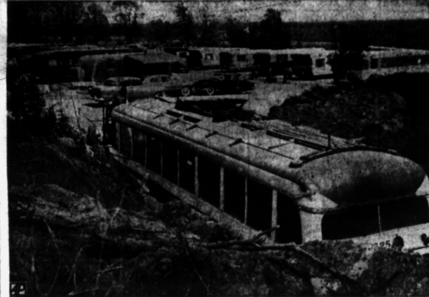
TORNADO SHELTER—A hole was cut in a bank at this trailer park on North Dort highway, north of Flint in the area hit by the tornado last June, and this old bus run into the opening. Now the bus will be tarred and covered to make a tornado shelter.
