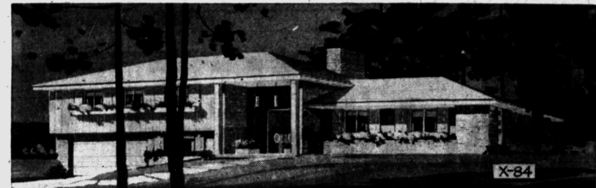
FOR TWO-CAR FAMILIES — There are nine big rooms in this handsome split level home. An outstanding feature is the im-
