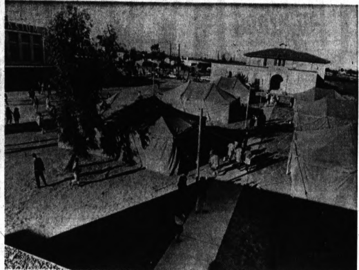
STUDENTS HAVE TENT CLASSROOMS —High School students walk past tents, used as classrooms, erected on school grounds at Calipatria, Calif. The two-story school building is empty, deemed unsafe by district trustees for the school's 320 pupils.
