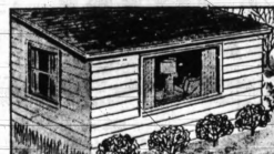
A ROOM ADDITION
