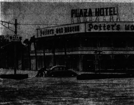
POWER IN THE REAR — A stranded car is pushed from a flooded street in downtown St. Augustine yesterday as heavy rains and high tides turned many of the town's streets into rivers.
