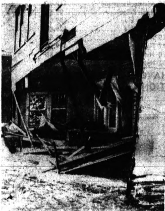
Jacksonville House Torn By Dora's Force
