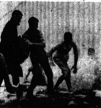
Try To Reinforce Jacksonville Seawall
