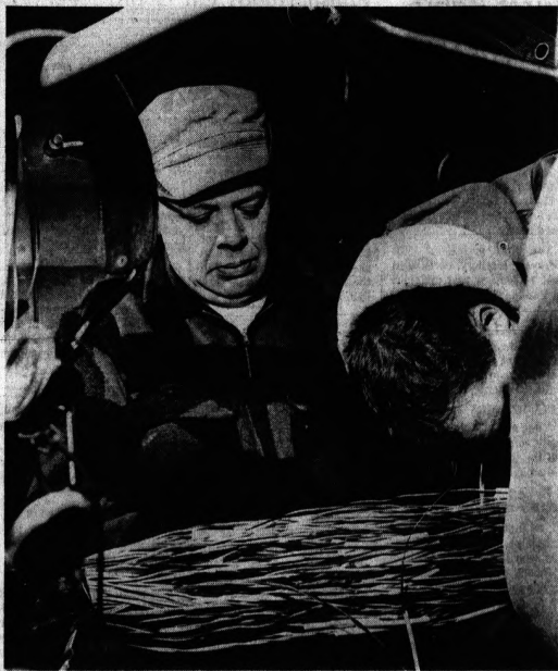
TEDIOUS WORK —Michigan Bell Telephone crewmen yesterday afternoon tackled a spaghetti-like mass of broken trunk lines to repair a five-hour service interruption in outside dial calls from the Oakland County area.
