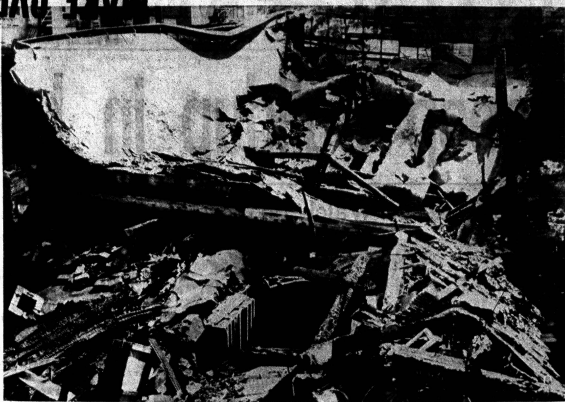
GUTTED BY FIRE — The ruins of the United Furnace Co.'s building at 21 Judson St. shows the intensity of the blaze which burned from 10 p.m. last night to 2 a.m. Although the roof and one wall collapsed, firemen escaped without injury. Total loss is estimated at $45,000.
