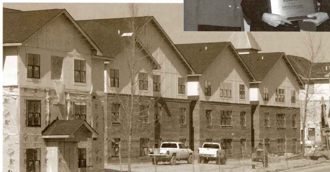
Above: University Student Apartments under construction.
