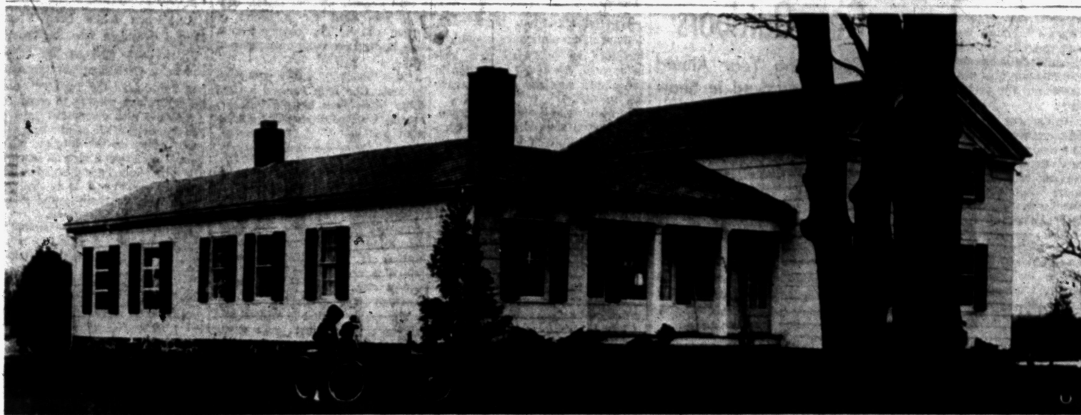
AGE-122 PLUS —Dr. and Mrs. Rockwood Bullard, Jr., selected this 122-year-old house at 8301 Foster Rd., Clarkston, for their family home and proceeded to do a renovating job. The original lines of the colonial house were preserved and by removing partitions the rooms became spacious. The foundation of the house is made of large
