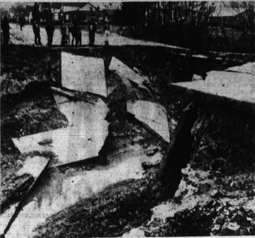
ROAD IN RUINS — A section of U.S. 2 in Ashland, Wis., 75 feet wide by 40 feet deep, was chewed away by a flood that raced through northern Wisconsin and Michigan's Upper Peninsula.
