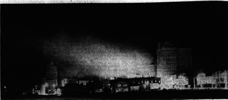
CITY BLAZE — Smoke from last night's fire at the Roosevelt Hotel drifts across downtown Pontiac. The 42-year-old structure was gutted. No deaths have been reported, although this morning some of the hotel's residents were reported missing.
