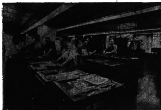
COMPOSITOR. This make-up man places your ad, according to classification in the chase—a heavy steel frame that holds a full page of type. When the page is complete, he locks the form to prevent the type from slipping. The page is prepared for the next process. The chase is wheeled to the...
