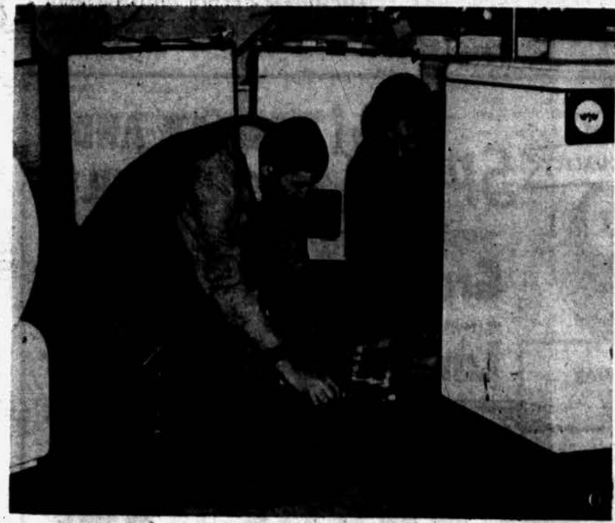
WHO SAID IT WON'T WORK? — Many families who discard household items as junk, would be surprised to find what the men at the Pontiac Men's Social Service Center of the Salvation Army can do to restore them to use. Here two men work over washing machines which will eventually end up for sale at the Center's Red Shield Store.
