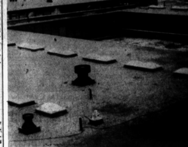
CLARKSTON'S NEW HIGH SCHOOL ADDITION — From the roof of the old Clarkston High School, the new rectangular addition and its pairs of plastic bubbles which are a new roof lighting device are visible. They provide the maximum of natural light in the classrooms, cafeteria, home economics department, music room and offices below.
