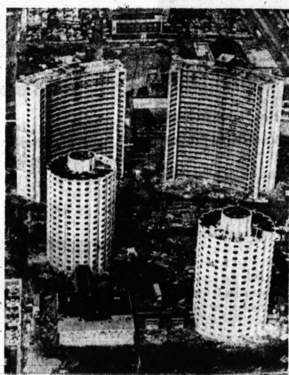
CHICAGO'S NEW LOOK—Two round and two gallery buildings go up south of Chicago's downtown district as part of public housing projects in the city. The towers will provide 784 apartments for the elderly. Gallery buildings will have 746 apartments for families.
