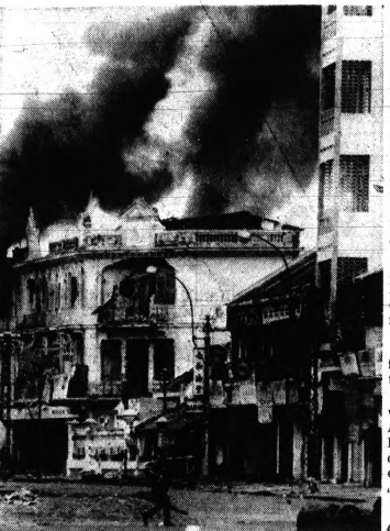
Saigon Building Burns After Rocket Hit
