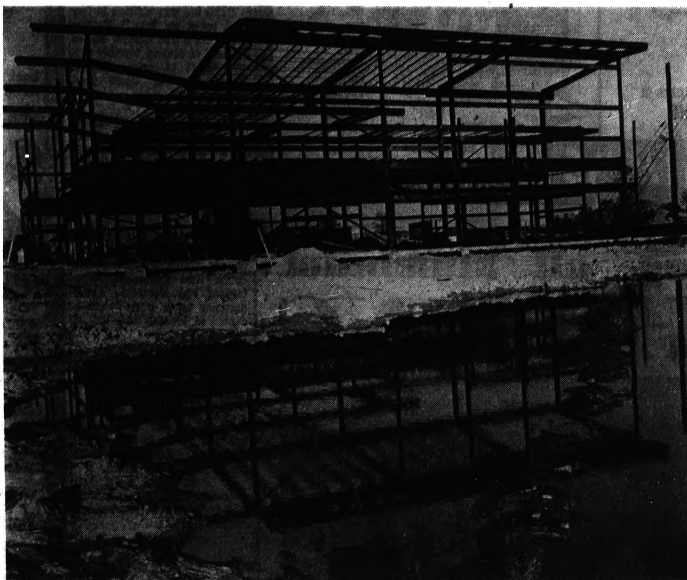
MALL NEWCOMER — While a construction strike has stalled progress on Bonwit Teller's new store in Troy, the frame is in place. The two-story structure, a part of the Somerset Mall Shopping Center, was scheduled originally for
