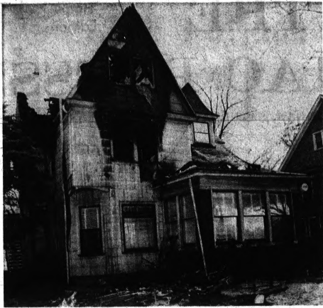
FIVE LEFT HOMELESS—Fire broke out early today at this four-unit apartment house at 263 Orchard Lake, leaving five persons without homes. Capt. Junior Deneen blamed faulty wiring originating in the second floor for the fire. He estimated "at least" $15,000 damage to the building and contents.
