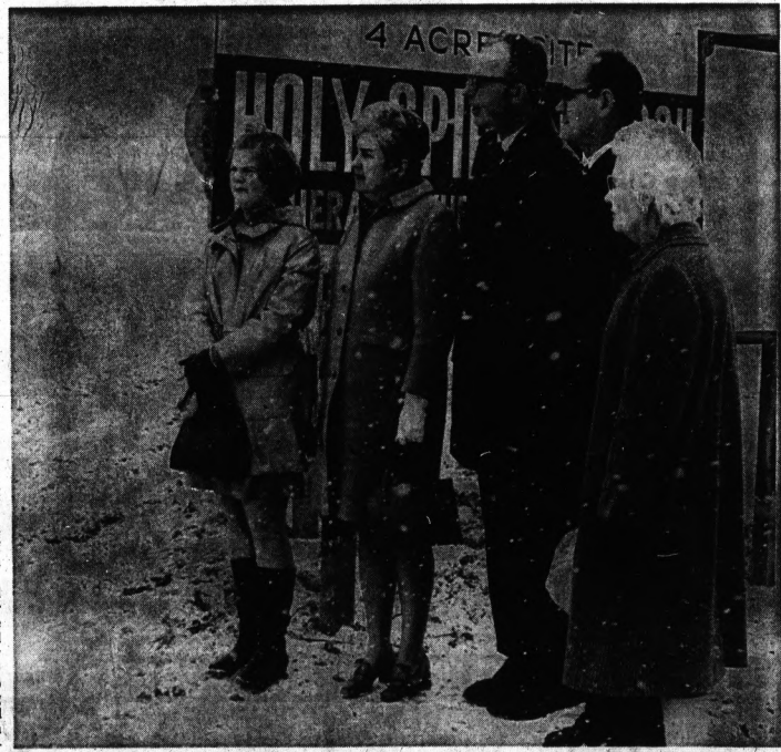
CHECK BUILDING SITE—"Let it snow" say the planners of the new Holy Spirit Lutheran Church when they meet on the building site this week to check the area. Shown are (from left) Chanda Zimmerman and her mother, Mrs. Harry
