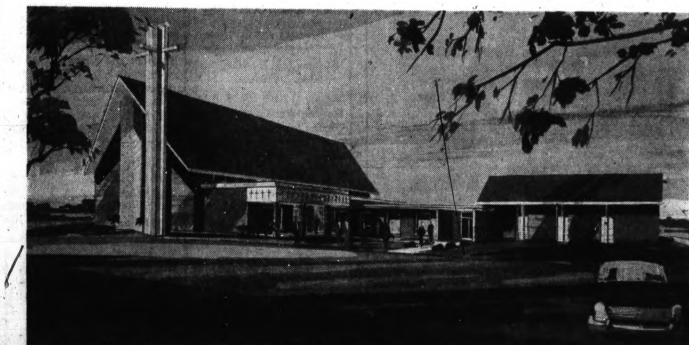
FIRST CHURCH OF GOD — The first unit of the First Church of God will soon be under construction. Located at 1333 Mt. Clemens in front of Galloway Lake, the cost will be near $100,000. Members of the building committee working
