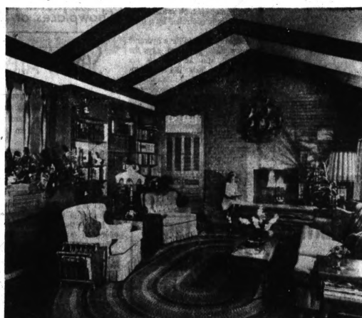
SLUMP BLOCK. —Resembling classic adobe in appearance only, sumptuous slump block fashions fireplace, provides decorator wall, and supports roof—all in one easy
