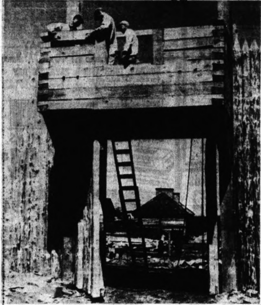
MASSACRE GATE — Workmen reproduce the massacre gate at restored Fort Michilimackinac at Mackinaw City. It was through the land gate that the original fort that Indians swarmed to massacre the British garrison in June 1763. The gate frames the British barracks restoration. The project probably will be completed by the July 4 weekend.
