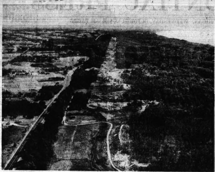
NOT NOW BUT SOON—This giant swath through the rich forests in Berrien County gives some idea what Oakland County will have to undergo when the State Highway Dept. within months begins work on the $34 million interstate freeway northeast of Pontiac. It will be part of Interstate 75 linking Detroit with South St. Marie. First contracts for work in the county will be let Dec. 7.
