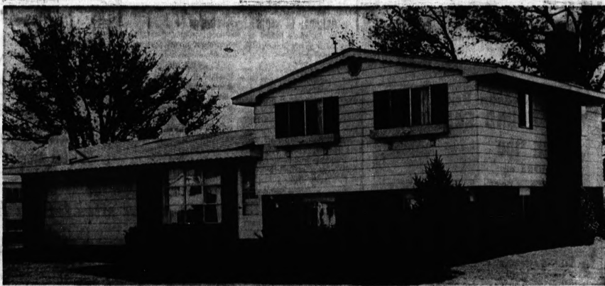
Used-Brick Trilevel Of Richard B. Royse Family Located On Ringwood Drive, Commerce Township
