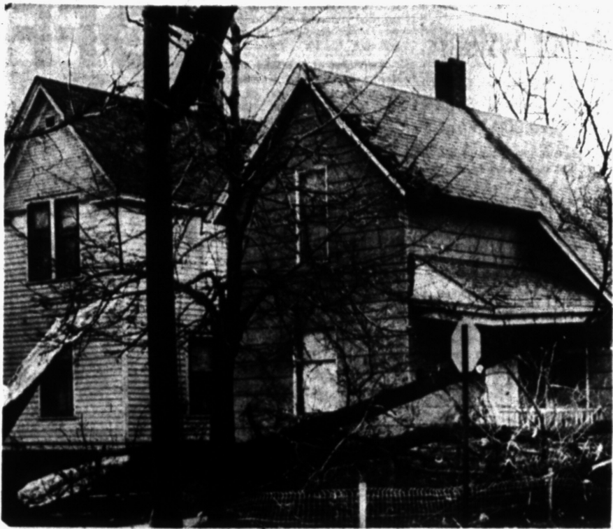
STORM DAMAGE —Near-hurricane winds yesterday downed this tree at the home of the Harold W. Gilberts, 66 Edison St. The trunk hit the roof and porch, causing an estimated $150 damage. No one was injured.
