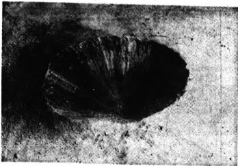
HOLE IN THE DESERT —Nuclear excavation experiment Cabrioleto blasted a 400-foot crater in Nevada with relatively little radioactive debris. But more and bigger tests will be needed before the bomb can be safely used for what it does best—making big holes. A five-bomb test is expected soon.
