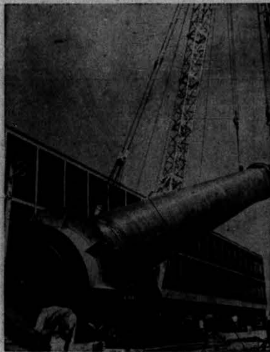
LOOK LIKE A GANNON? — What appears to be a cannon is nothing more than a giant stainless steel chimney, 77 feet long, being raised to its permanent mooring at Bloomfield, Conn.
