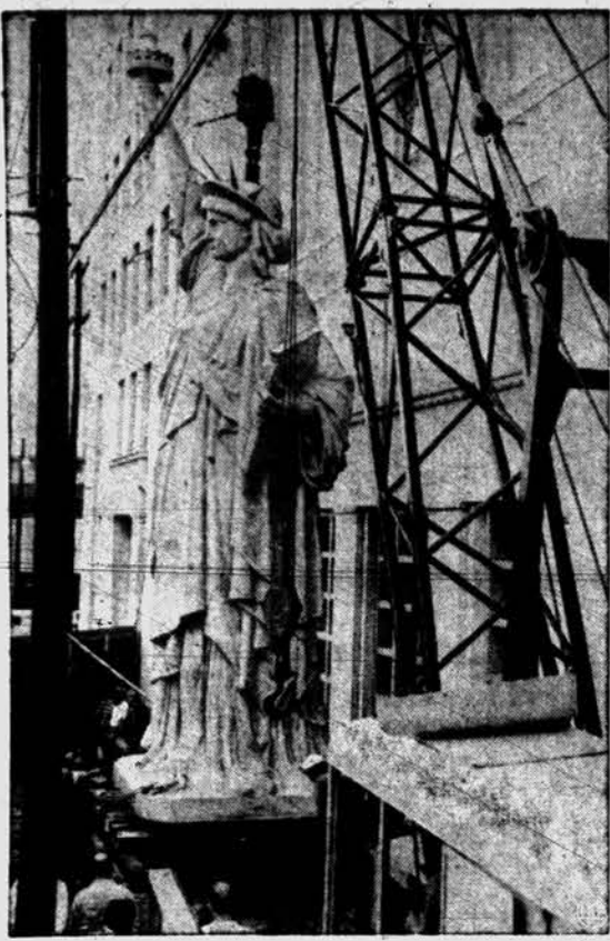
LIBERTY RISING — What at first glance looks like the Statue of Liberty in unfamiliar surroundings is actually a one-fifth-size replica of America's famous Lady. The 31-foot, 20,000-pound bronze statue is being hoisted to the top of the Liberty National Life Insurance Building in Birmingham, Ala., where its gas-fired torch will shed light 184 feet above the city. Like her big sister in New York Harbor, Miss Liberty was made in France.
