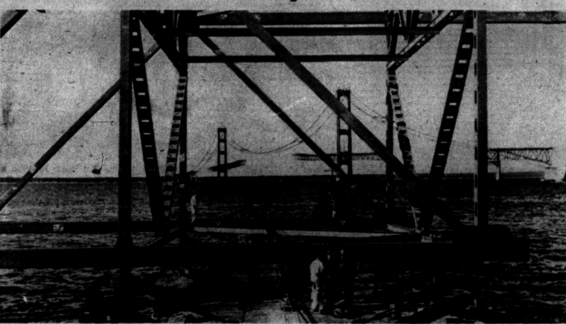
MAKING READY — The Mackinac Bridge is framed in the distance by steel members of this pre-assembled section, called a stiffening truss unit, being towed to the construction site. Floating
