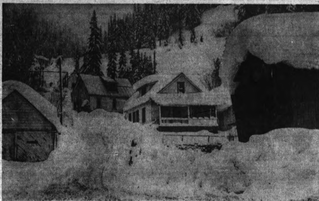
PLENTY OF SNOW — Houses and sheds at the head of Burke Canyon in north Idaho groan under the weight of heavy snow piled up this week. Measuring stations about one
