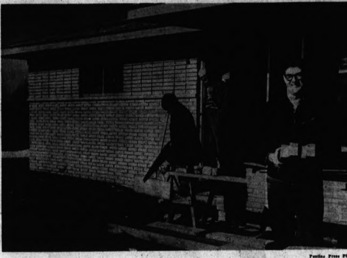
BUILDING PARSONAGE —Laying bricks at the new parsonage of the First Church of God on the 16 acres of land purchased for a new church on Mt. Clemens Street near Galloway Lake are (from left) Lester McFarland of 73 Trill St. and Jacob Goltzy of 830 Coughlan St. Pastor E. D. Johnson stands in the doorway of the home. In September two dwellings were given the church to tear down for lumber. Men, women and children turned out to raze the buildings and pull nails from lumber. Freeman Brandt, contractor and member of the church, is doing the building with volunteer help.
