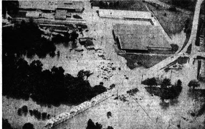
FLOOD CUTS HIGHWAY — This aerial photograph shows how the Blue River flood has cut off U.S. 71, a main entrance to Kansas City from the southeast. A bridge over the river is at the lower left near 8th Street. The large building at the center is a warehouse of the John Deere Implement Co. Ruins and winds caused by Hurricane Carla have caused property damage and five deaths in Kansas.
