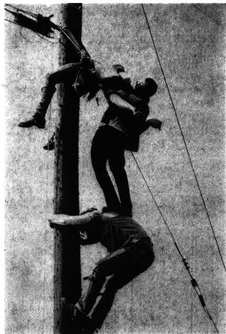
DRAMATIC RESCUE ATTEMPT — Charles Whited, 21, of Nanty Glo, Pa., was electrocuted yesterday when he touched a 2,400-volt power line while installing a television cable. Tom Streams of Indiana, an ambulance service employee, tried to revive Whited with mouth-to-mouth resuscitation while standing on the back of another man from the TV cable company, Ronald Viney, 22, of Twin Rocks.
