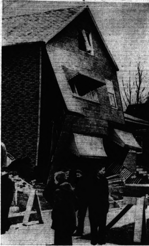
SOMETHING SEAMS WRONG — A tornado which struck Chicago's South Side redesigned this frame home. The front wall took on a bulge at the seams but the building remained pretty well intact. Many other buildings in two storm-battered areas remained standing, but they were damaged beyond repair. The destruction figure was pegged at $5 million.
