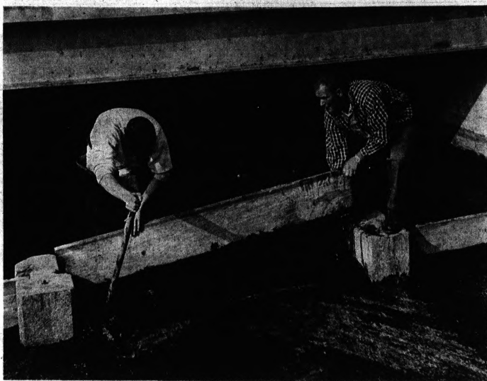
LETTING THE WATER OUT — Lake Orion Department of Public Works employees raise the M24 dam gates in a process which will eventually lower the water level in Lake Orion by 42 inches. Paint Creek will catch the spill-over. A
