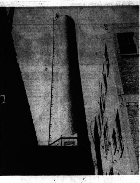
REAL Y PIECEWORK — Because other bricks prevent working equipment from piling down this 150-foot smokestack, Jim McTeer, the dot on the top, is taking it down one brick at a time. He removes about 500 bricks per hour, and figures he has a steady job for at least six weeks.
